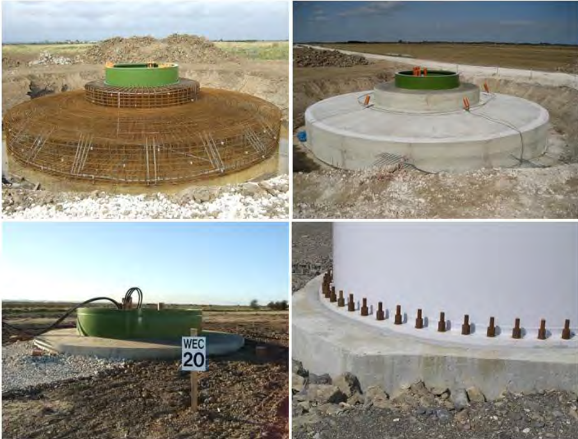
Figure 2.6-1: Example of Turbine Foundation Construction Stages Photos courtesy of Enercon
