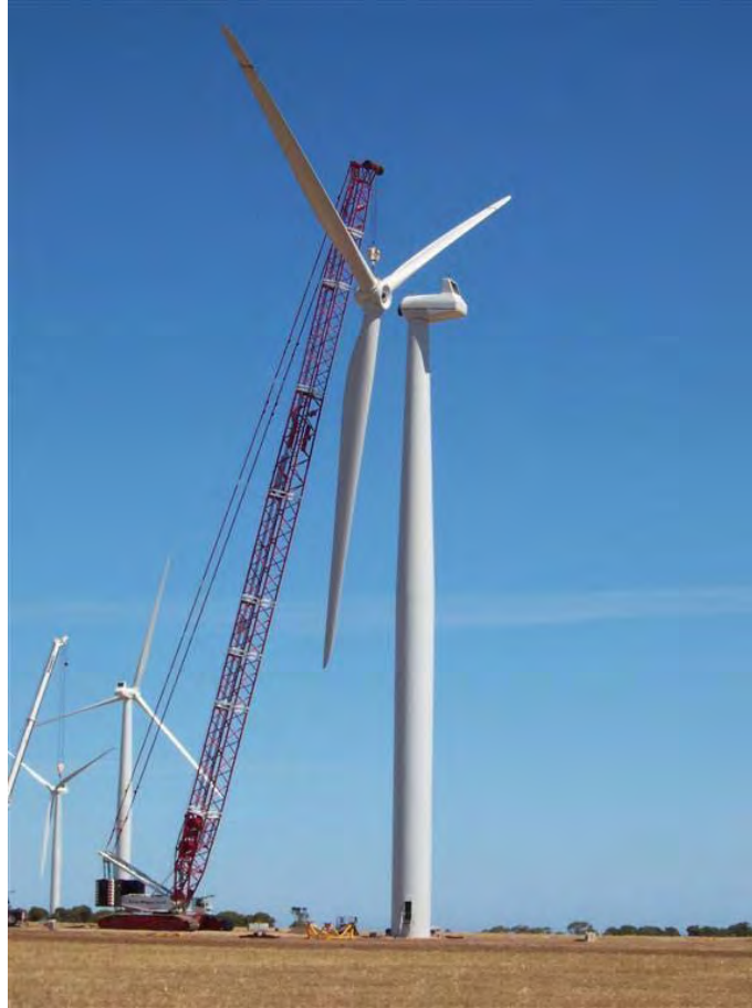
Figure 2.5-3: Example of a Crawler Crane Source: KR Wind
